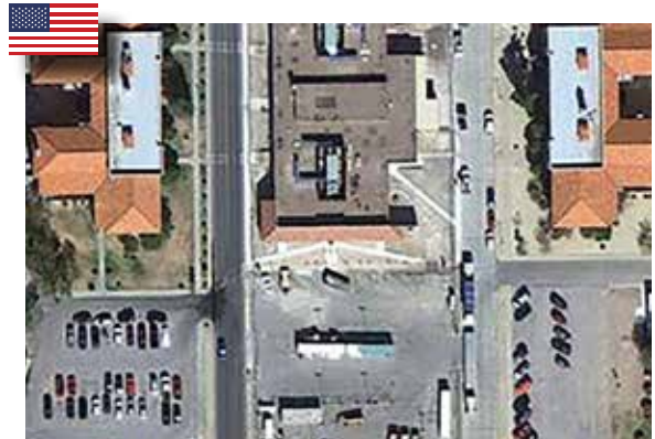
Fort Bliss Army Base United States | Coolerado | Stand-alone Cooling
