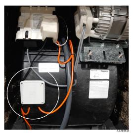
Drill 2 holes to suit the 16mm glands provided in the MobileMAX Tank kit and fit the glands.
