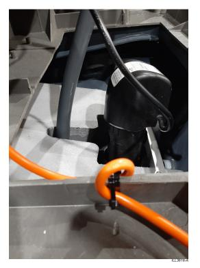
From the cooler packout kit, locate the 1.0m lead with an IEC plug at one end.
