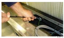
From the inlet side of the cooler, pull the cable through the conduit.
