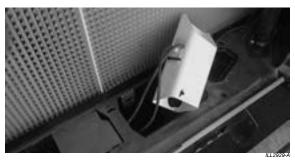
Withdraw (and insert) the enclosure assembly on an angle as shown above.
