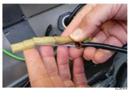
Tape the three terminals together in a staggered formation to make it easier for the cable to be pulled through the conduit without snagging.
