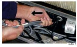
Pull the bundled cables through the conduit from the inlet side of the cooler. Do not force the cable as damage to the connectors may occur. If the cable becomes stuck, push it back through and try re-taping the connectors.
