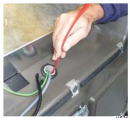
• From the electronics enclosure side of the cooler, feed an electrician's cable chasing snake through the conduit.
