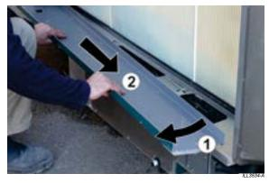
Unscrew the utilities mount and pull out bracket with chlorinator attached.
