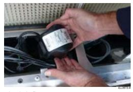
· Pull out the drain Pump.
