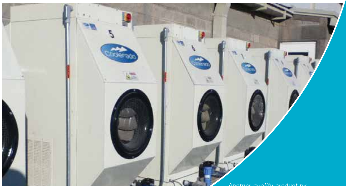
Kellogg's Food Processing Plant at Mexicali, Mexico
